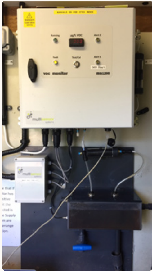
A picture of the unit installed in the outbuilding. The unit controls a sluice gate which diverts flow away from the reservoir in the event of contamination.
