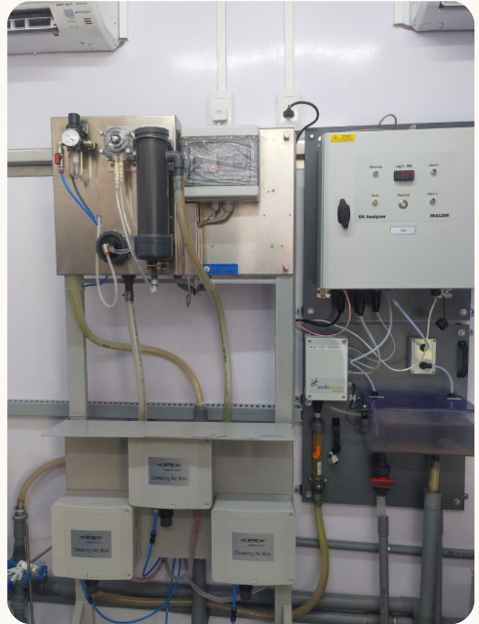
MS1200 and filtering system installed side by side
