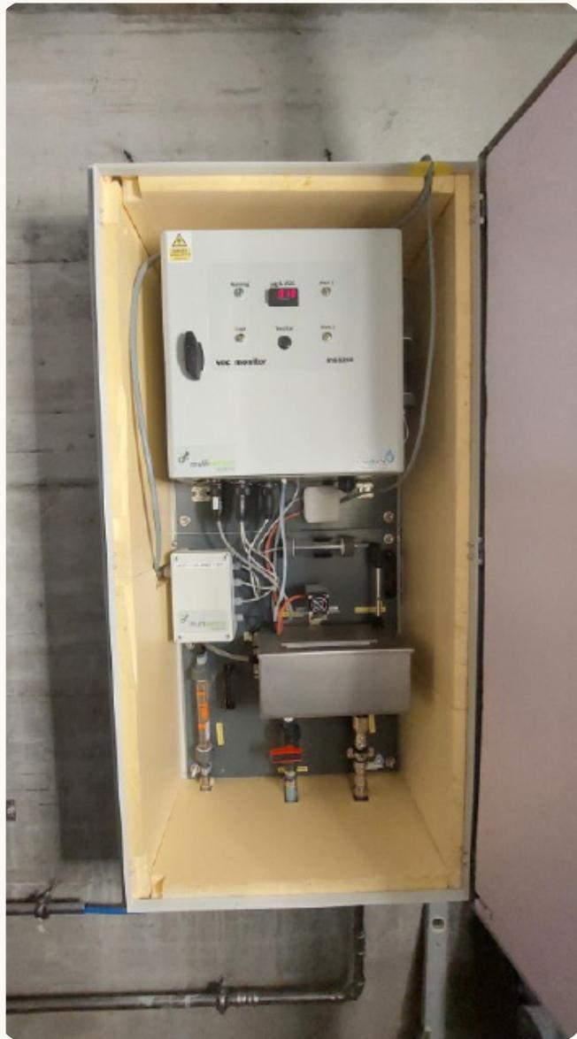
**MS1200 installed into a cabinet with internal insulation; the insulation was the best way to ensure that the instrument was protected**
