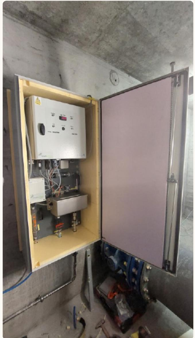
**The water is taken directly from the main line using the existing pressure and goes back into the spring from a return pipe.**
