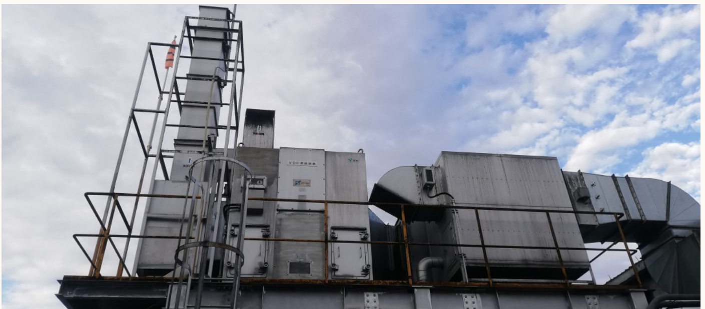
Full view of the VOC removal unit; one of the main issues was to climb over the tower several times a way to take a sample. The sample usually was taken from an opening on the side of the main tower.
